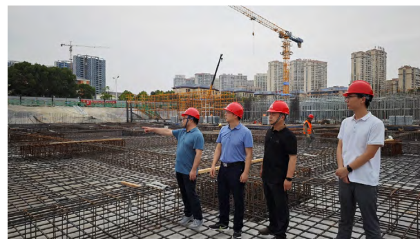
The safety inspection team inspecting a project site in Lushan
