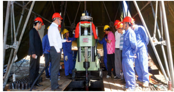
Geological exploration drilling site in Zimbabwe
