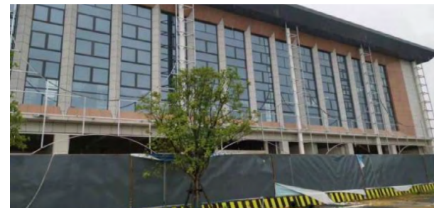
Door and window installation project site
