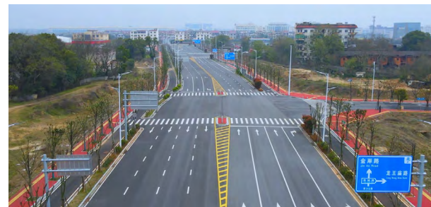
Municipal road project
