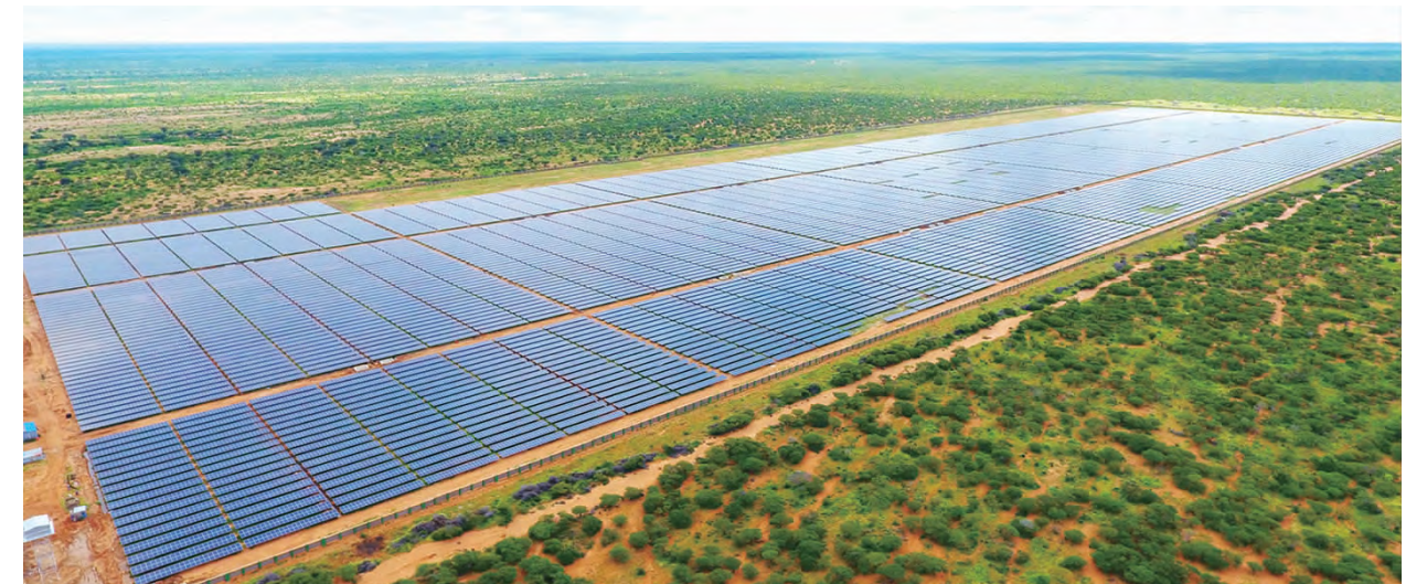
The 50-MW Solar Power Plant Project in Garissa, Kenya, is expected to generate 76.467 million kilowatt-hours of power annually over its 25-year operational period. This will help reduce carbon dioxide emissions by approximately 64,190 tonnes per year and save around 24,470 tonnes of standard coal.
