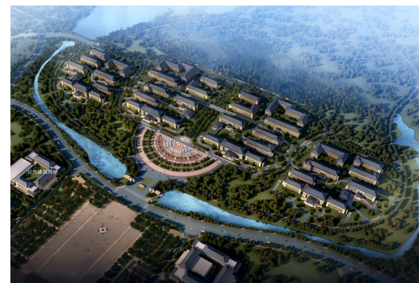
Jiangxi Provincial Party and Government Offices Relocation Project
