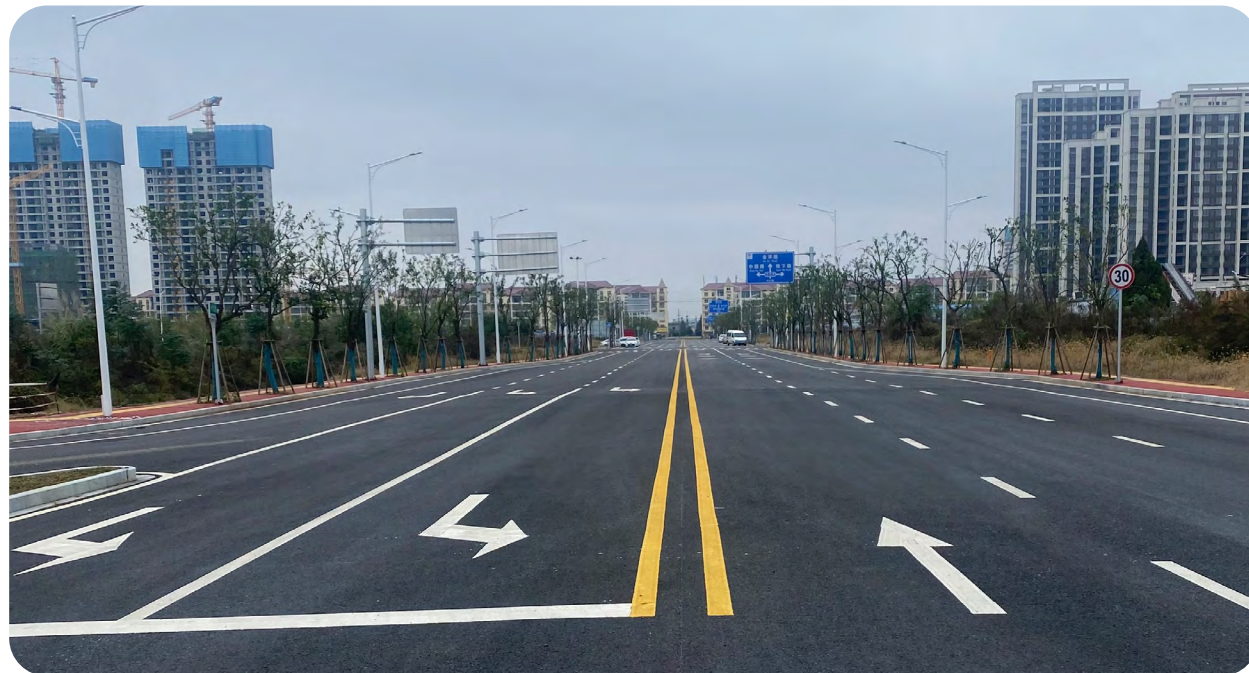
The municipal road construction of the Heli Port-City Integration Project in Zhangshu received high praise from the client, supervisor, and local government for its excellent quality and zero-accident record
